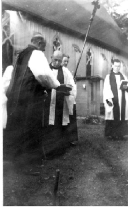
The Ground Breaking
